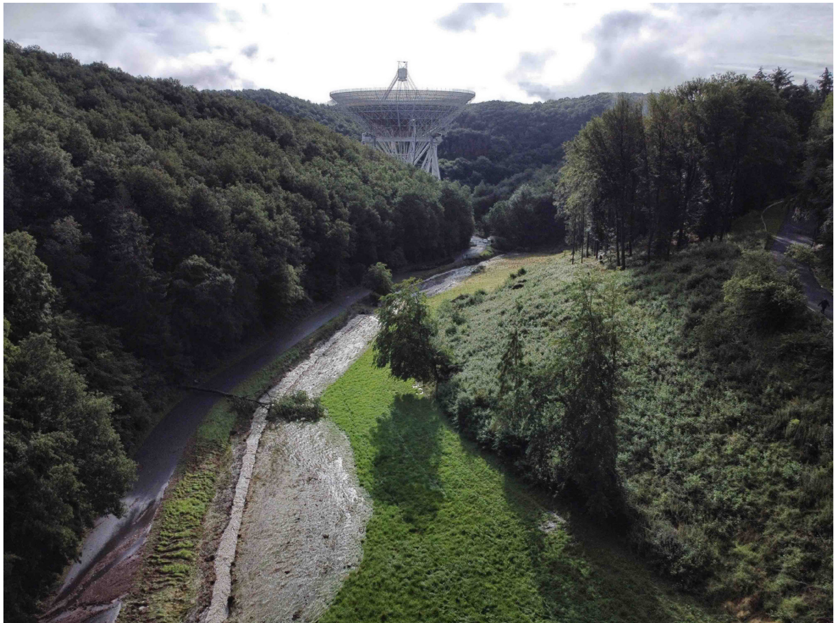
The picture shows the access road to the 100 m radio telescope Effelsberg with the Rötzelbach running parallel to it. Normally a rather narrow trickle, it led to flooding of the road and the adjacent meadow during the heavy rainfall of July 13-14, 2021.
